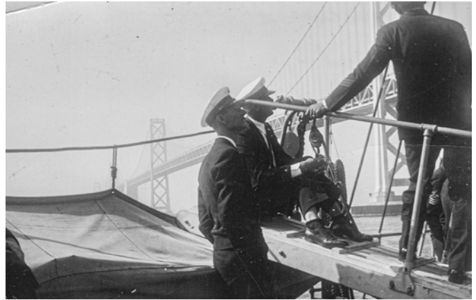
Passing under the San Francisco - Oakland Bay Bridge. 16 Oct 39
