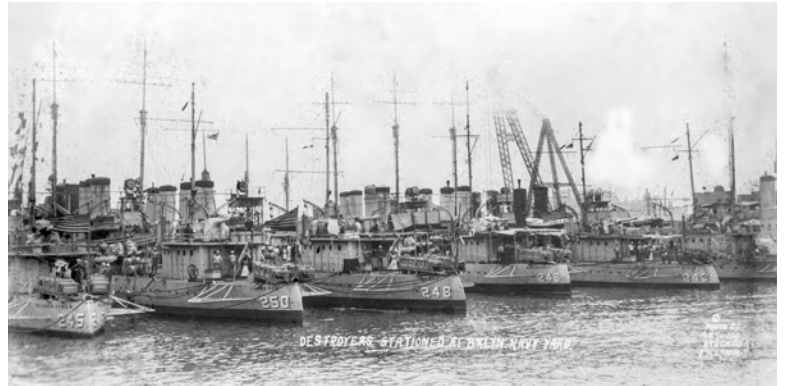
Destroyers at Brooklyn Navy Yard. From left to right: USS Ruben James (245), Lawrence (250), Barry (248), Bainbridge (246), Sands (243), all were commissioned in 1920 and 1921.
