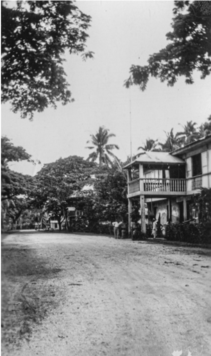
Left: Municipal Building Provincial Road Dapitan, Mindanao P.I. 28 Apr 38
