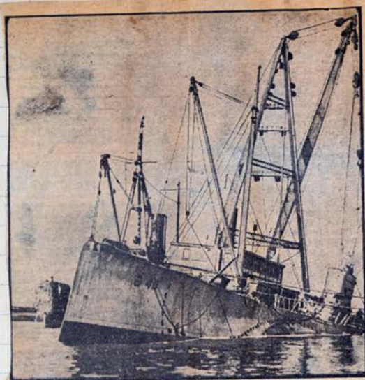
Floating derricks are shown raising the submarine S-48, which went to the bottom, off Bridgeport, Conn., in December, 1922. It sank in shallow water.
